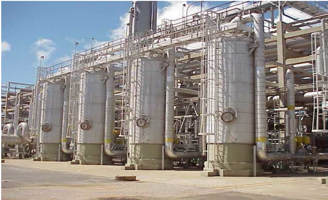
fig. 1.10 (Tamices moleculares)
