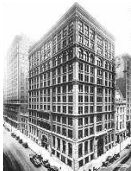
Foto: Home Insurance Building . Demolido en 1931.
