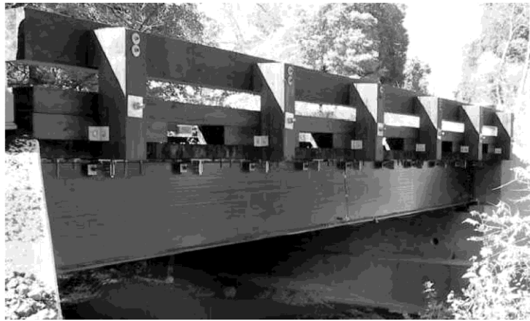
Figure 1.9 FRP DWB girders on Dickey Creek bridge.
