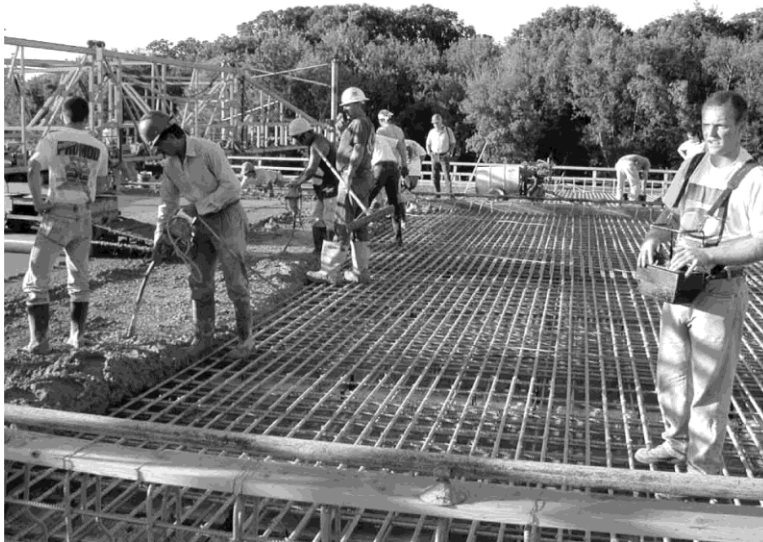
Figure 1.4. Bridge deck slab with a glass FRP top mat being poured.
