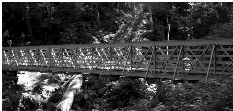
Figure 1.8 Light-truss pedestrian bridge pultruded structure.
