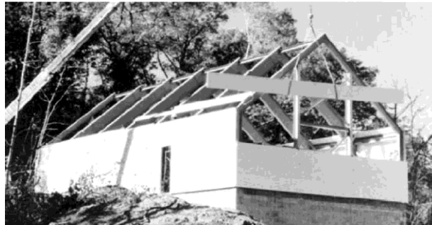
Figure 1.6 FRP frame structure under construction.
