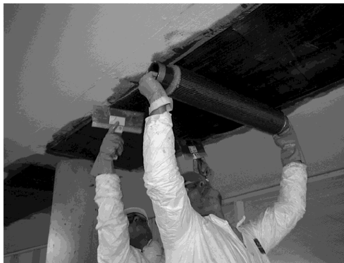
Figure 1.5 Installation of a carbon fiber fabric sheet.
