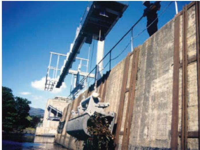
Figura 93. Hydro Bosker Raking Machine (Fuente: Brackett Green)
