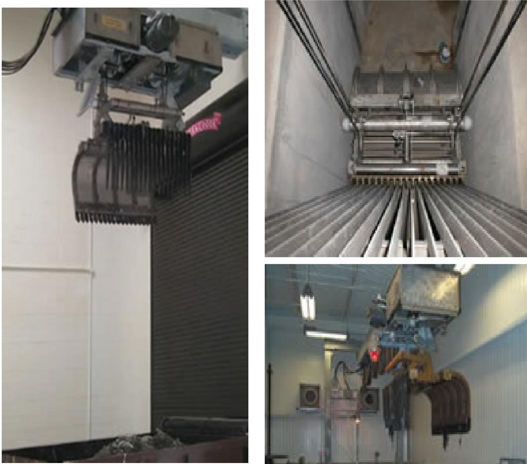
Figura 92. Sewage Bosker Raking Machine (Fuente: Brackett Green)
