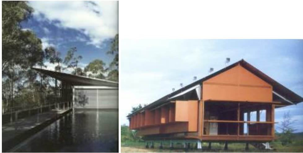
Figura 51: 1. Simpson-Lee House. Mount Wilson.1994 2. Marika-Alderton House.1994 .Imágenes tomadas de Glenn Murcutt a singular architectural practice.
