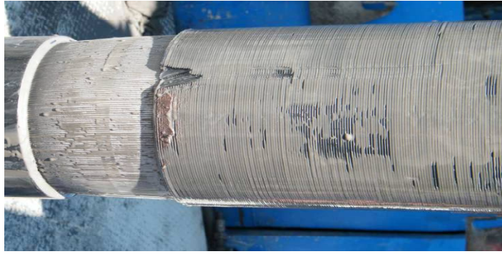
Figure 3.5. Damage on Rubber Sleeve
