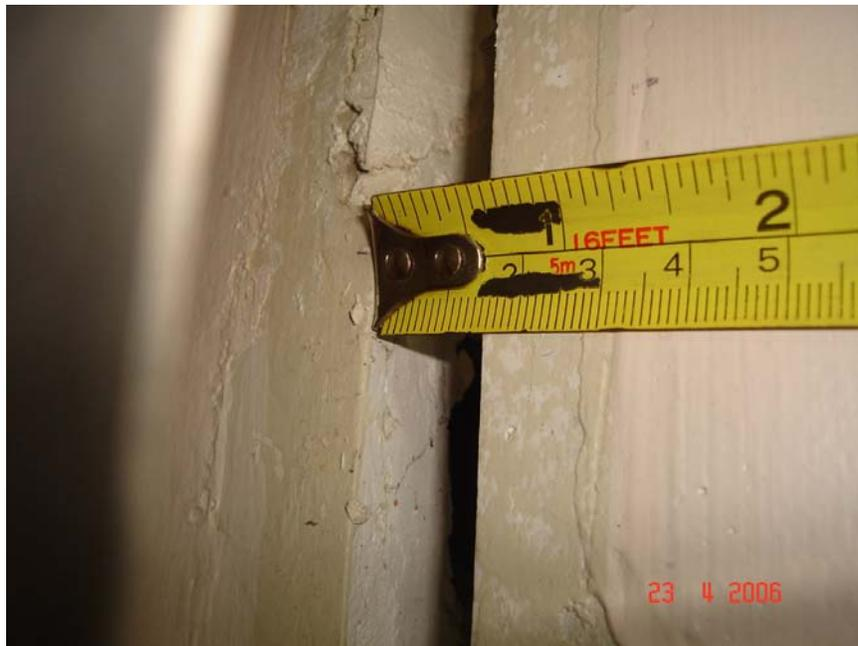
**Detalle Junta Pared – Sin Platina. MIV – MV. Piso 1.**
